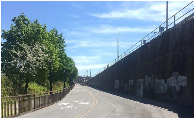
The existing retaining wall is imposing to pedestrians.
