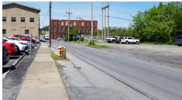
Existing sidewalk along Newell Street
