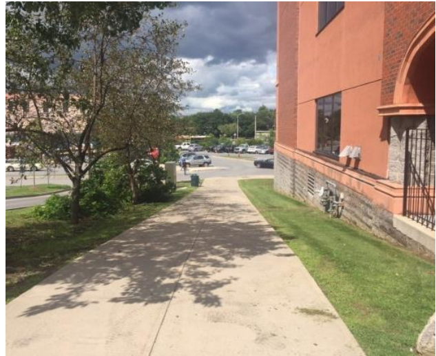
Existing western sidewalk connection to the JB Wise Parking Lot
